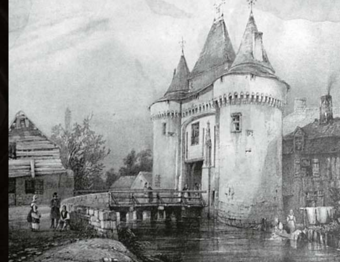
Saint-Julien gate, before the replacement of the wooden lintel by a stone arch towards the end of the 19 th century, by J. Jacottet, lithography Lemercier.
