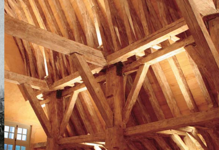
Oak rafters restored in 2006-2007 in the covered market.
