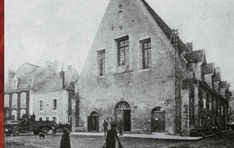
Place de la Lice and the market hall, between 1914 and 1918. The current statue of Saint Louis is not in the niche above the central bay.
